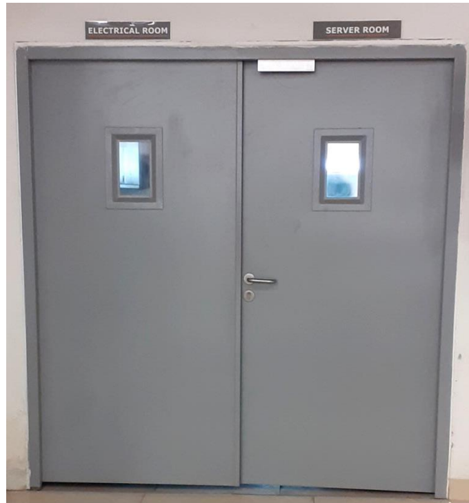
Electrical and Server Room
